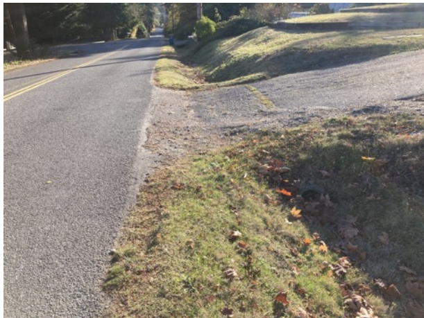
Example of Existing Conditions
